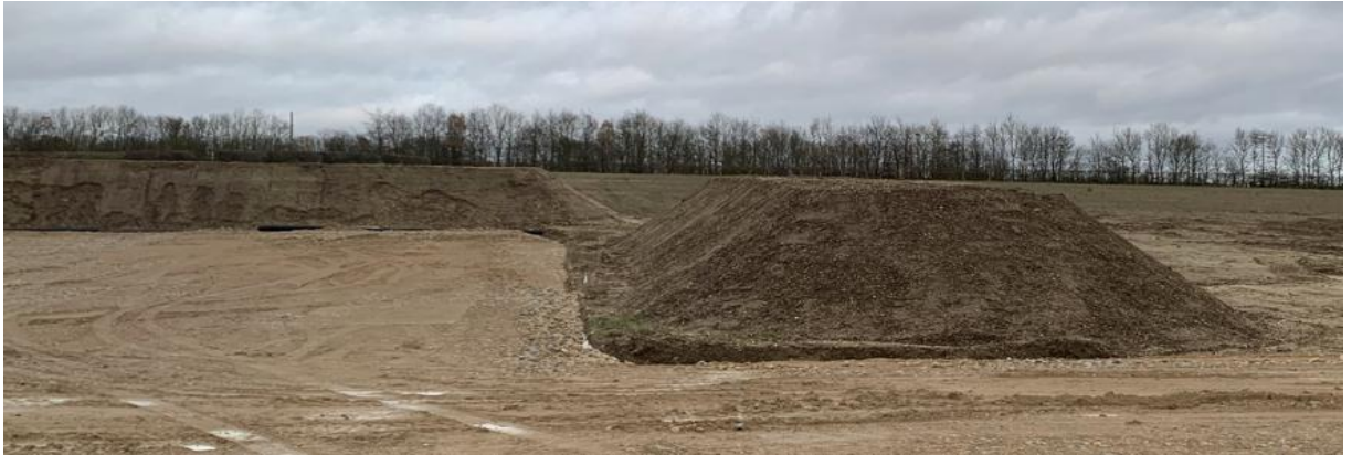
Photo 16: Topsoil Storage Example (Elsham – Lincoln Pipeline)
